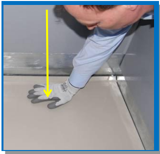
5. Ensure that base (Plastic or Steel) inside the unit is firmly pushed down.
